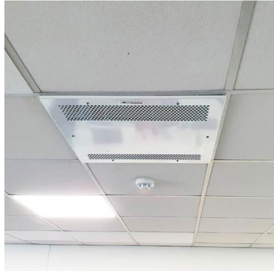
K7 600 Logistic Company Sales Office
